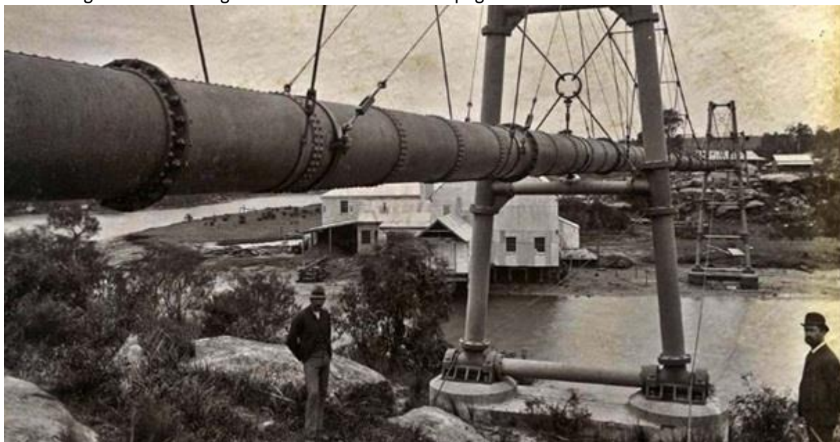
Source: http://dictionaryofsydney.org/image/43779 Titled - Construction of the suspension bridge carrying water pipes across the Lane Cove River 1890. By Blomfield, Harold Arthur. Contributed by Private Collection (Courtesy of Charles Blomfield, Wagga Wagga)
