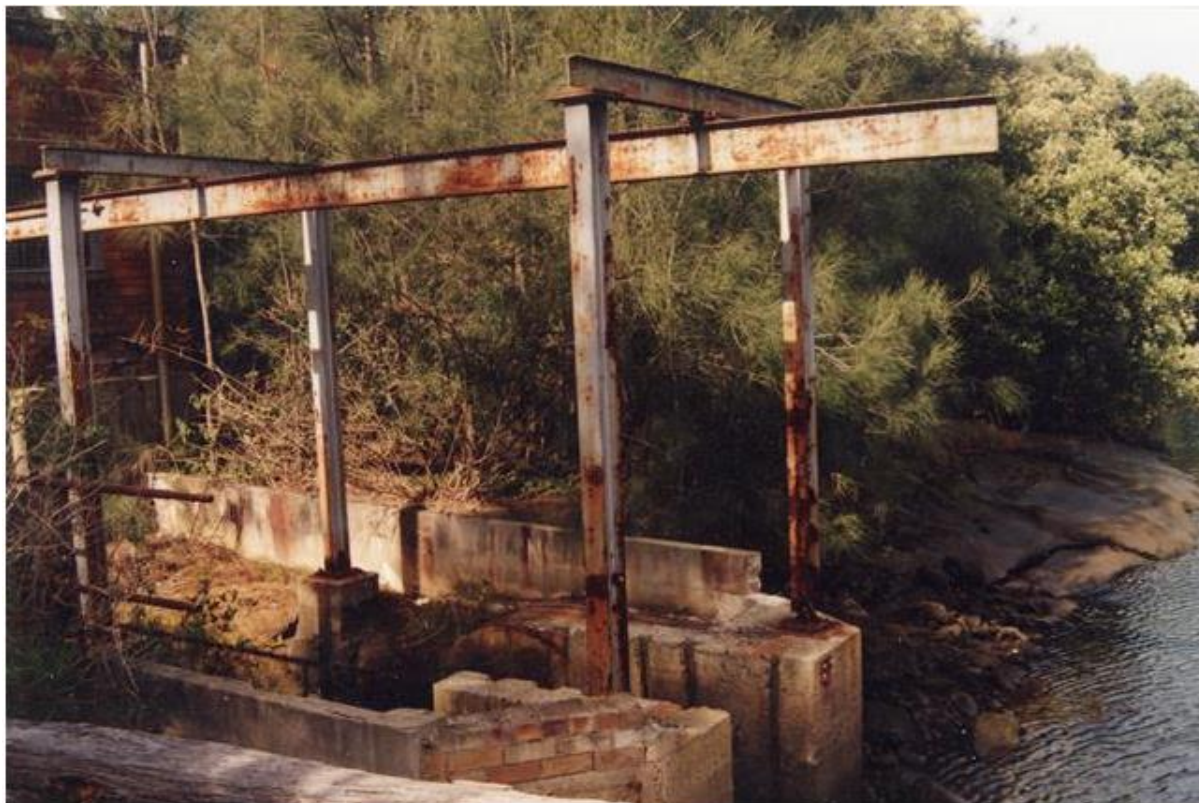
The photographs feature the CSR Chemicals saltwater pumphouse and adjacent wharf
