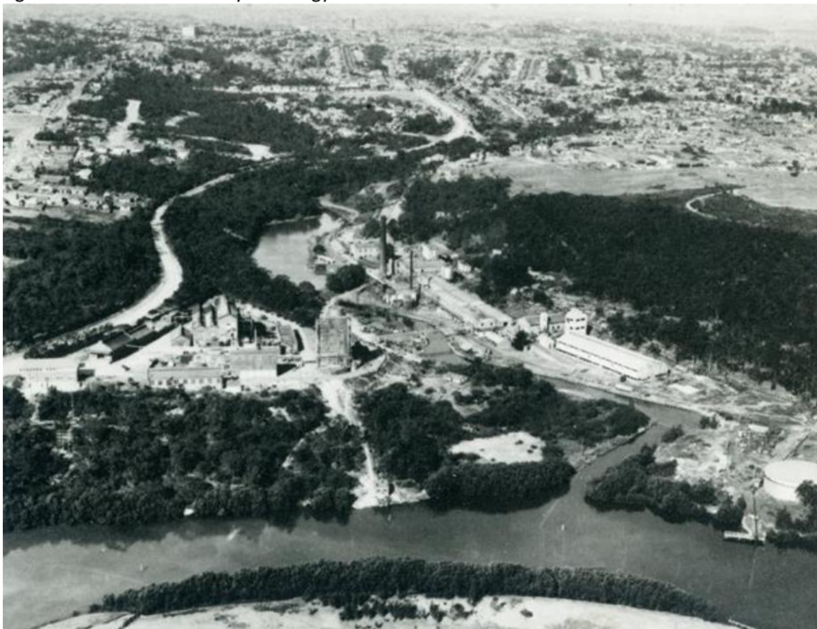
Above: Lane Cove River at bottom of picture. Stringybark creek leading up to dam. Molasses Tank and jetty to the right of Stringybark Creek. Water pump house to left of Stringybark Creek.
